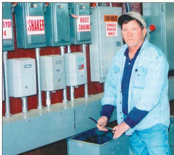
Local electrician Ronnie Coats installed the capacitors.
