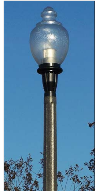
Acorn-type fixture w/clear globe
