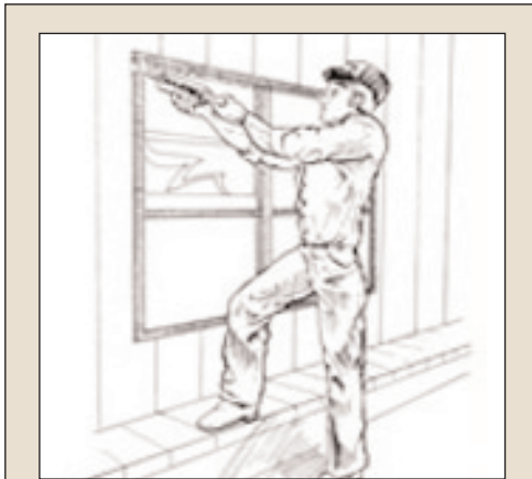
Above: Inspect windows and apply caulking to seal air leaks. Below: Caulk or plug holes around faucets with proper material.
